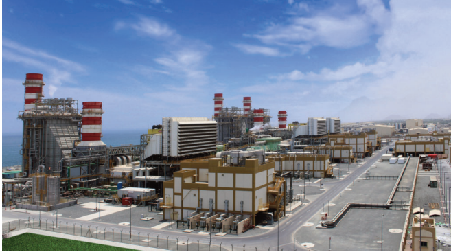
Fujairah F3 Power Plant
