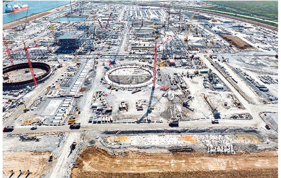
Construction advances on Sempra's Port-Arthur LNG terminal
