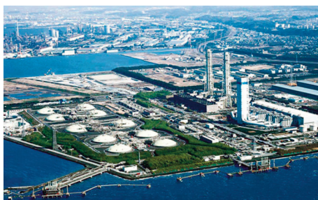
Nghi Son LNG-fuelled power plant in central Vietnam
