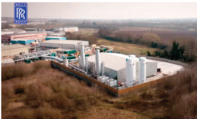
Gas engine power plant with CO 2 recovery
