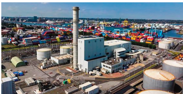
Dublin Bay power station
