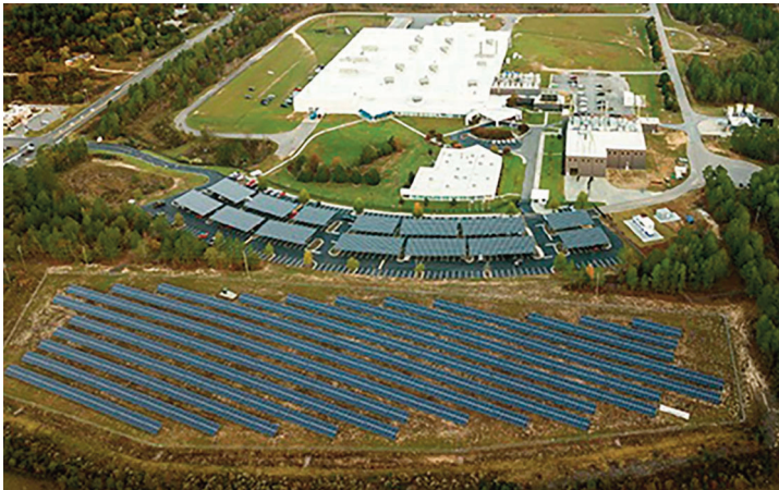
mtu Series 4000 factory at Aiken, South Carolina
