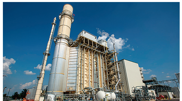
View of Middletown Energy Center
