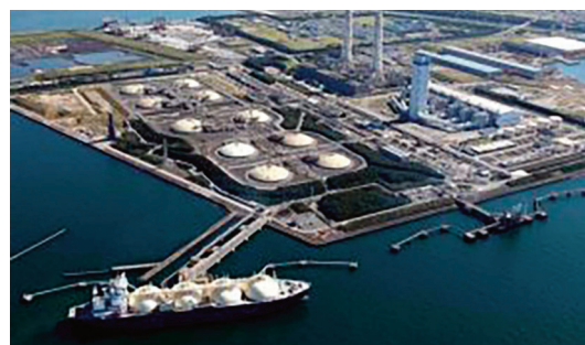
JERA LNG terminal with adjacent power station
