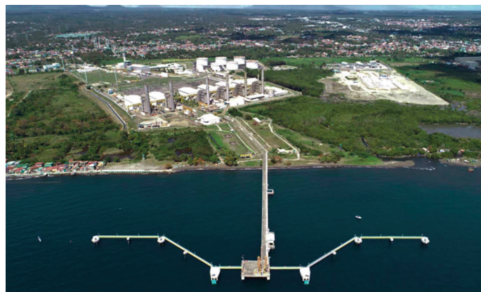
Bird's eye view of BW Batangas FSRU
