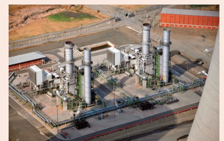
Secunda power plant
