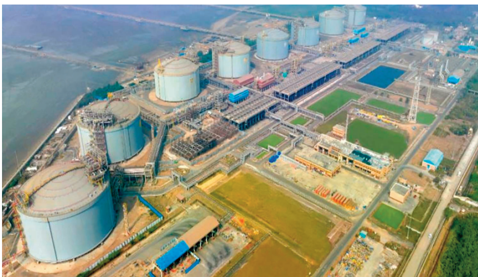
Dahaj LNG terminal is being expanded
