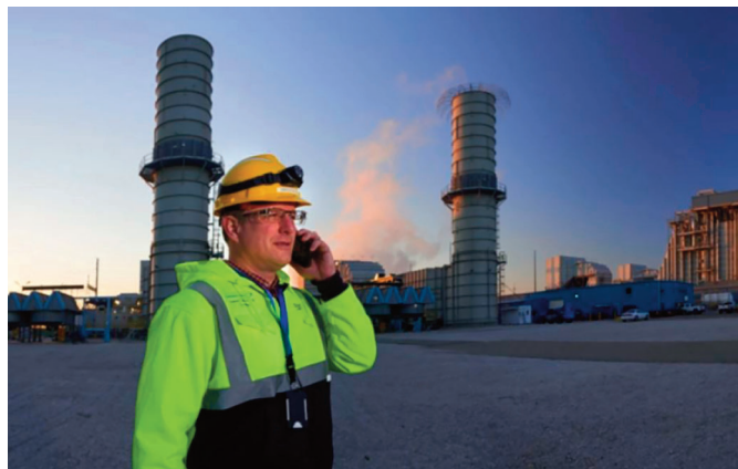
Zeeland Generating Station
