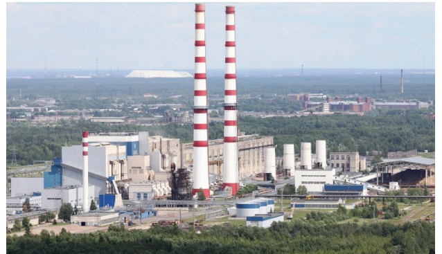
Enefit's Narva Balti Power Plant complex
