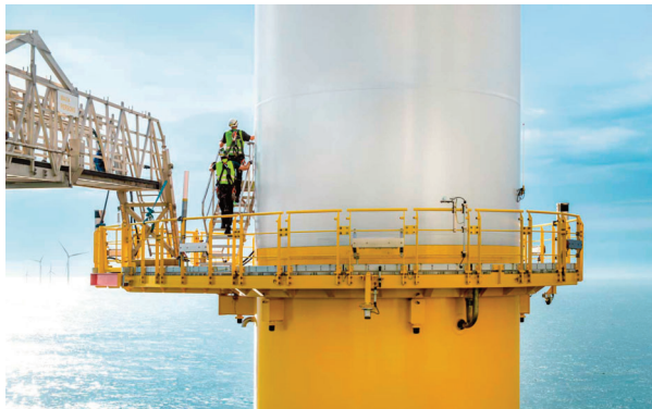
Close-up of offshore wind park
