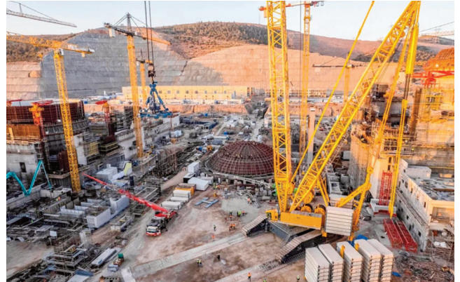
Works to install inner containment dome of Akkuyu reactor
