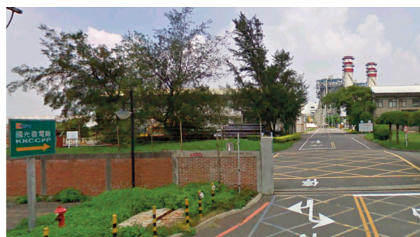
Kuo Kuang power plant in Taoyuan City, Taiwan
