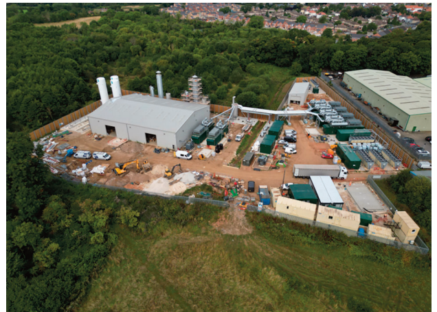
Site view of Rhodesia project in Nottinghamshire
