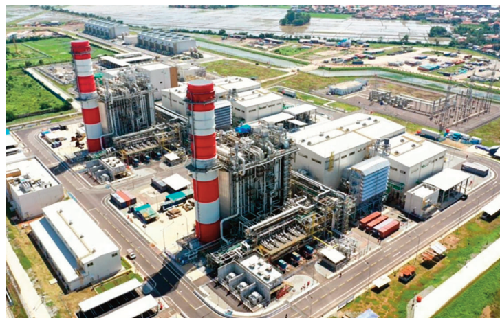
View of Jawa1 gas-fired IPP
