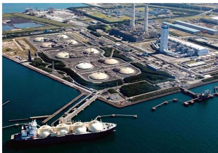
Futtsu LNG terminal and power plant at Tokyo Bay
