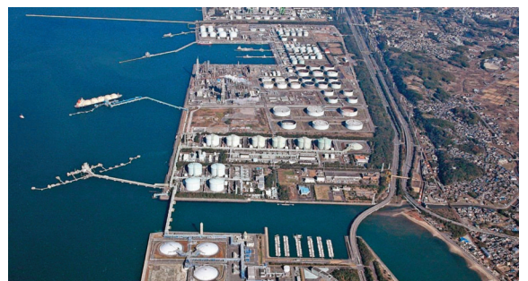
Bird's eye view of Chita thermal power station
