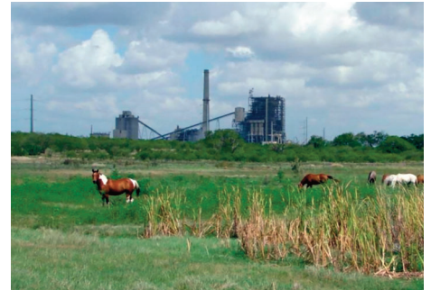
San Miguel Electric Coop's plant on farmland
