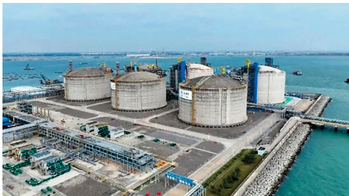
PipeChina’s Beihai LNG terminal that received sanctioned Russian LNG
