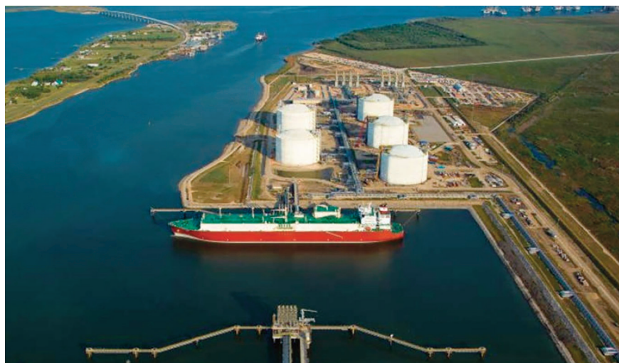
Venture Global's CP2 terminal in Cameron Parish, Louisiana
