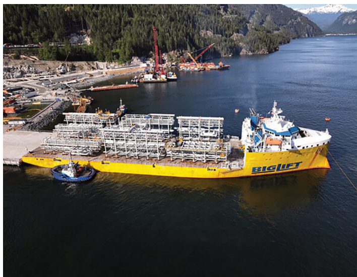
The first modules arrive on site
