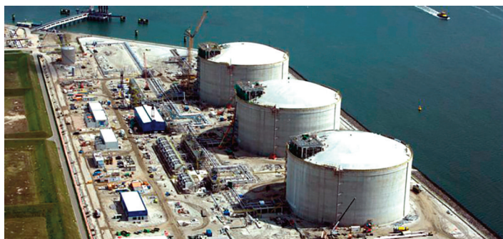
Three of Gate terminal's storage tanks seen under construction
