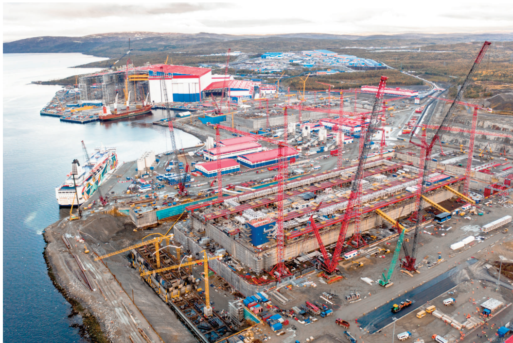
Murmansk is the location of a large module construction site for Russian oil and gas projects
