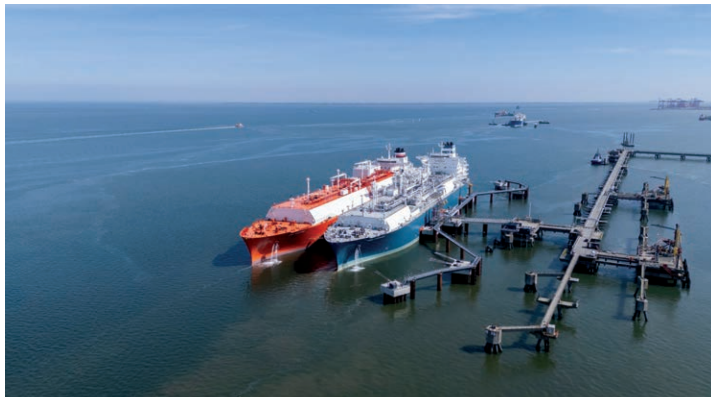
Deutsche Energy Terminal's (DET) Wilhelmshaven facility
