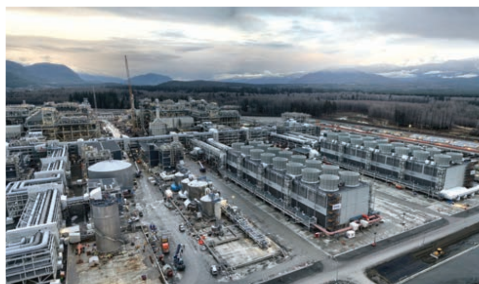
Construction is well advanced at the LNG Canada terminal
