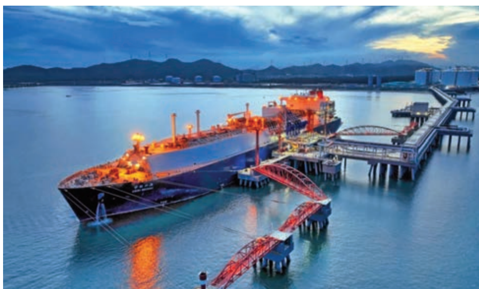
Huaying LNG terminal, developed by Sinopec in Guangdong province
