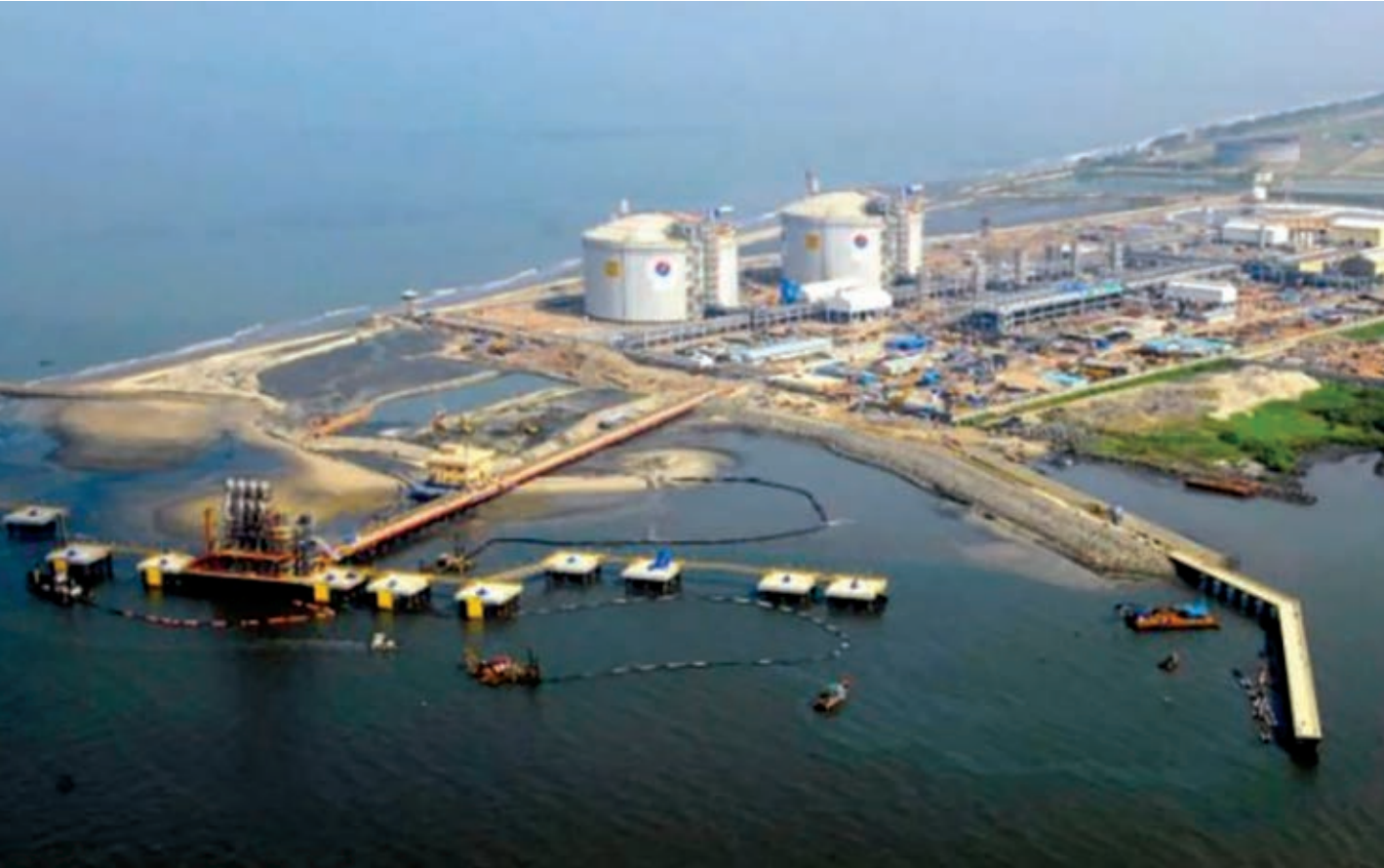
Bird's eye view of the Chhara LNG import terminal in India's Gujarat state
