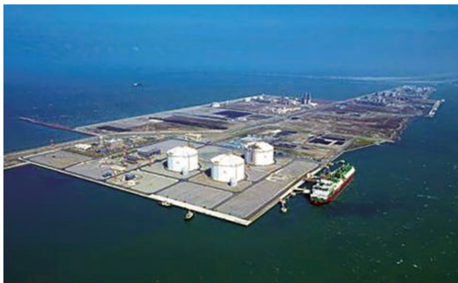
Bird's eye view of Taichung LNG terminal (under expansion)
