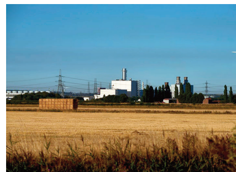
Keadby 2 site in North Lincolnshire
