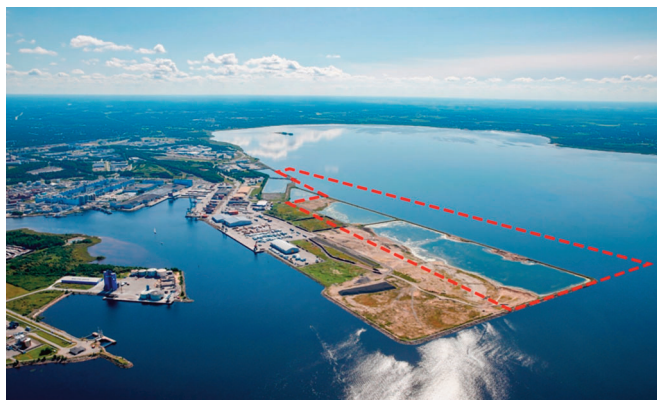
Site of Verso Energy's projected synfuels plant at Oulu Port
