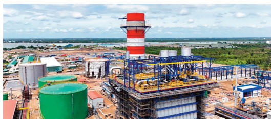
Nhon Trach 3 & 4 power plant
