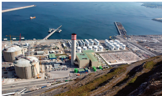
BBE at the port of Bilbao
