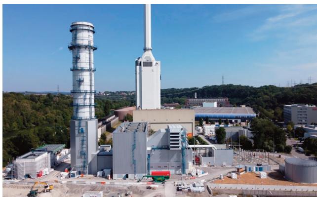
EnBW's new Marbach grid-stabilisation plant near Stuttgart
