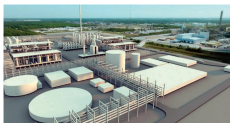
Render of ExxonMobil's facility in Bayton, Texas
