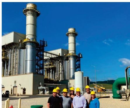
DOE NETL team at Cane Run power station
