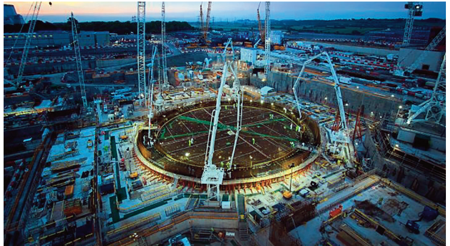
Construction progresses at Hinkley Point C
