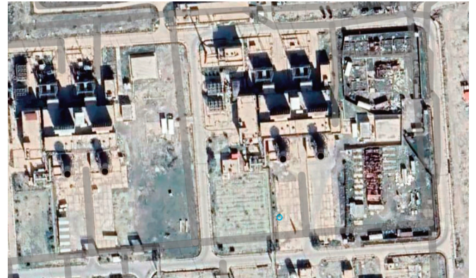
Birds eyes view of Baiji power station
