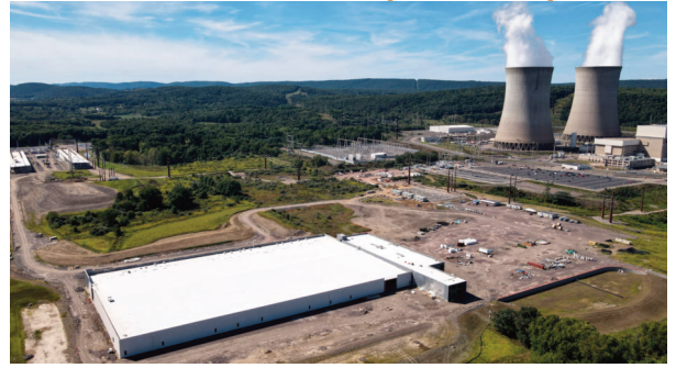
Data center next to Susquehanna nuke
