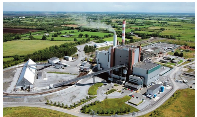
Shannonbridge OCGT will be built on land of the West Offaly Power Station
