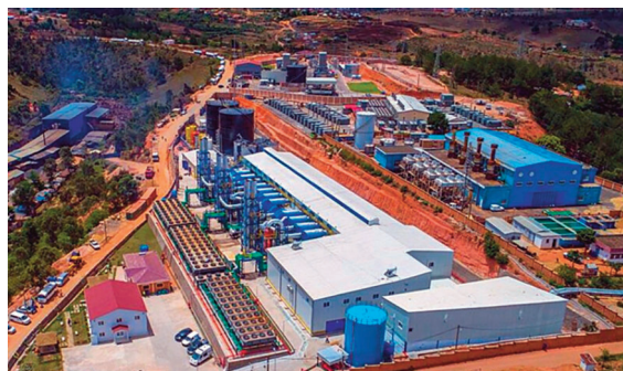
Site of Saint Louis CCGT in northern Senegal
