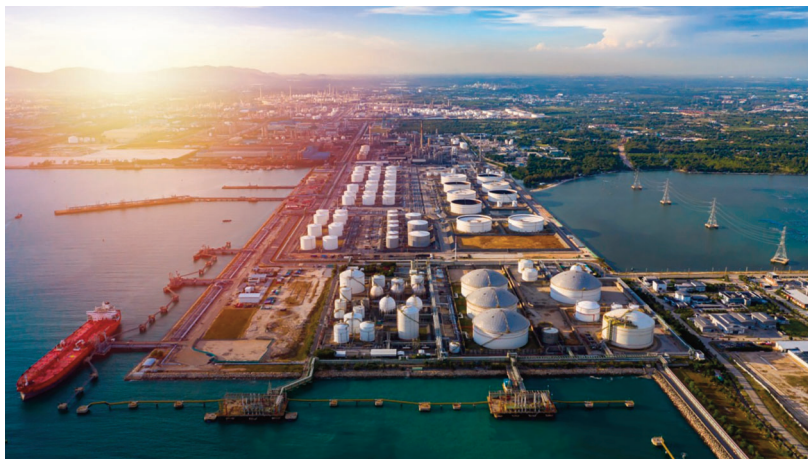
Bird's eyes view of Chhara LNG terminal
