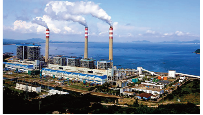
View of the 5,000 MW Yangxi power plant in Xitou Town, Guangdong
