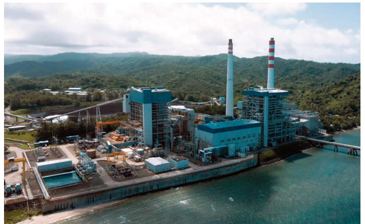
Quezon coal power plant (460 MW)
