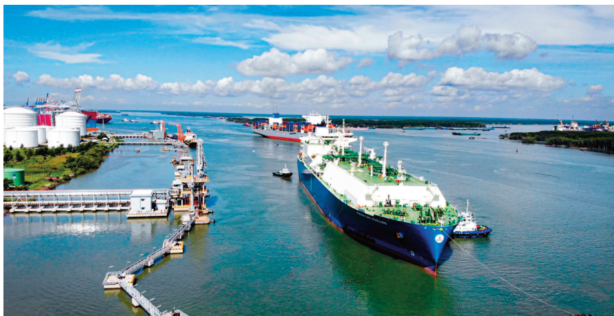
View of PV Gas' Thi Vai import terminal in Vietnam
