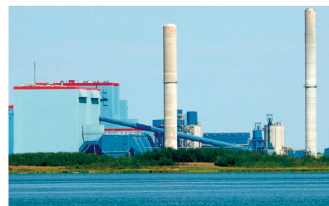
Genesee Generating Station near Edmonton
