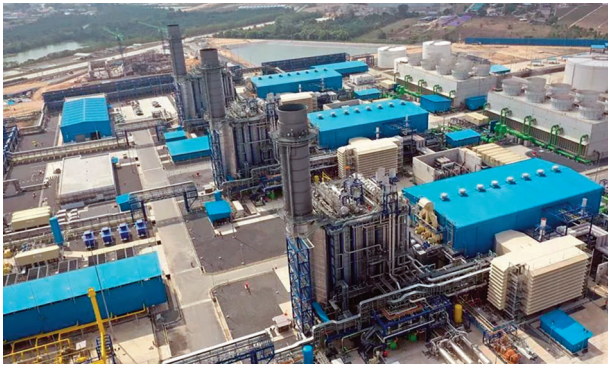
Rayong combined-cycle plant on Thailand's east coast
