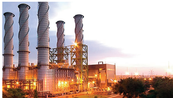
NTPC's Jhanor Gandhar gas power station
