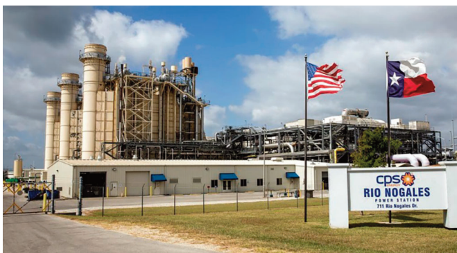
CPS's Rio Nogales gas peaking power plant
