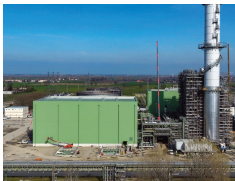
Tavazzano and Montanaso power plant
