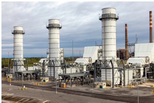
Three new units at Paradise plant
