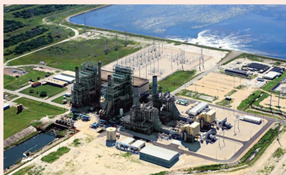
Barney Davis power plant in ERCOT
