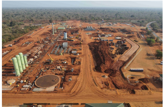
Construction work for Temane power station
