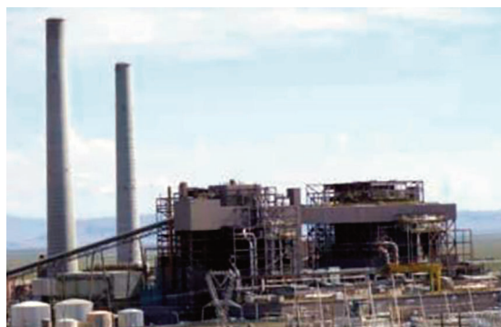
View of North Valmy Generation Station
