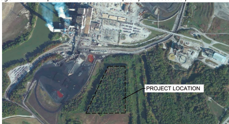
Location of battery at AES' Petersburg Generating Station
