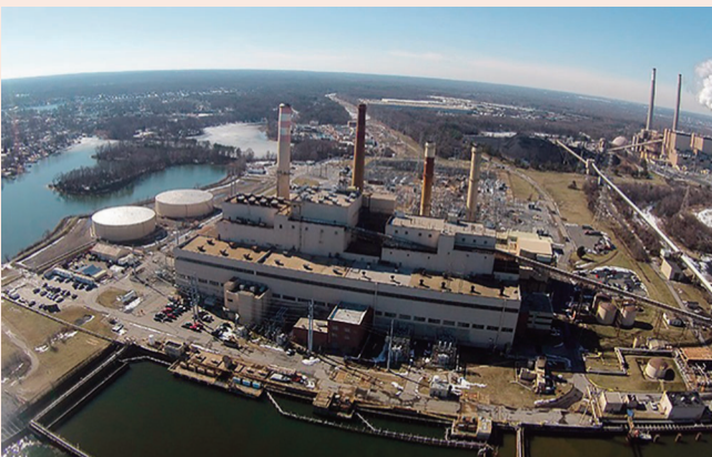
Talen's Wagner Generating Station
