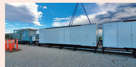
Delivery of PowerTitan BESS
