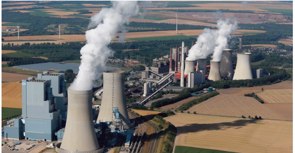
RWE's Neurath C lignite power unit
