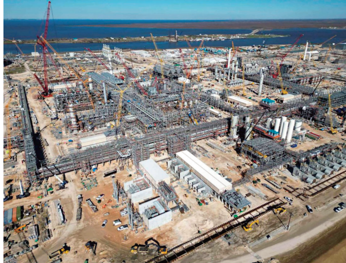
Construction progresses at Golden Pass LNG in Texas
