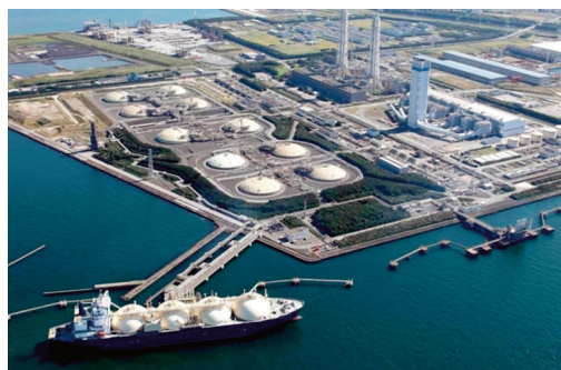
Futtsu LNG regas terminal and power plant at Tokyo Bay
