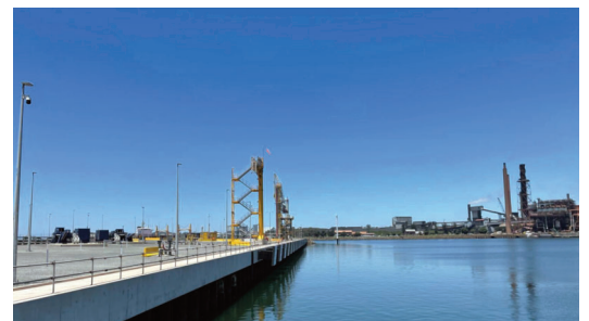
Port Kembla's LNG receiving terminal completed
