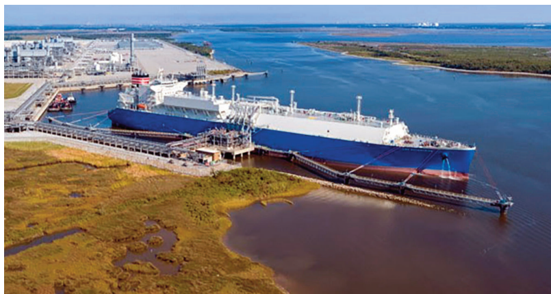
TotalEnergies is to supply LNG to Botaş
